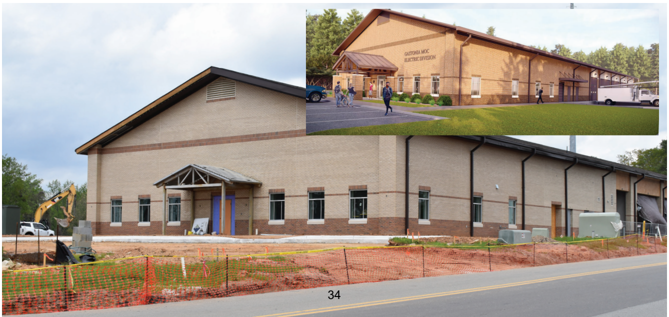
Construction for Electric Division Municipal Operating Center
