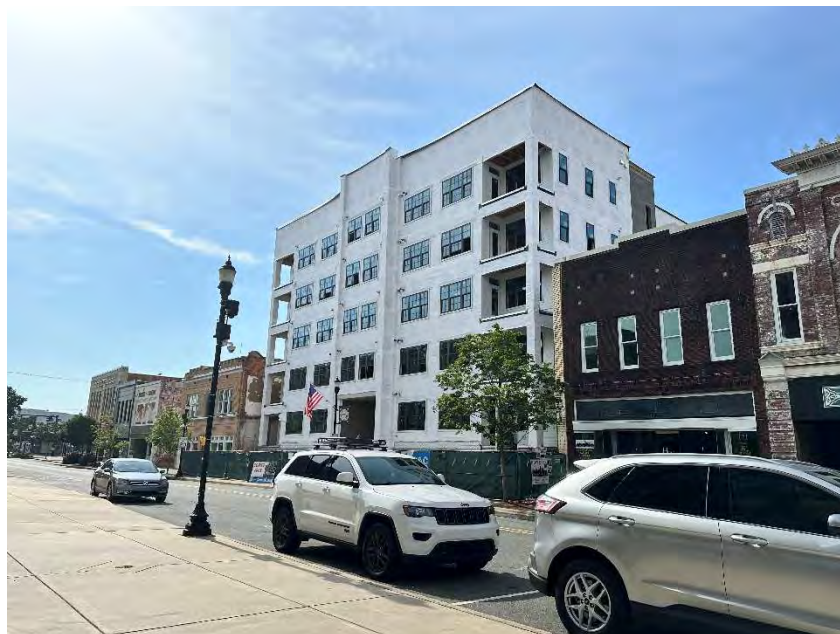
Center City Crossings Under Construction in Downtown Gastonia
