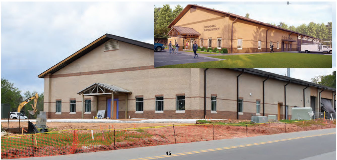
Construction for Electric Division Municipal Operating Center
